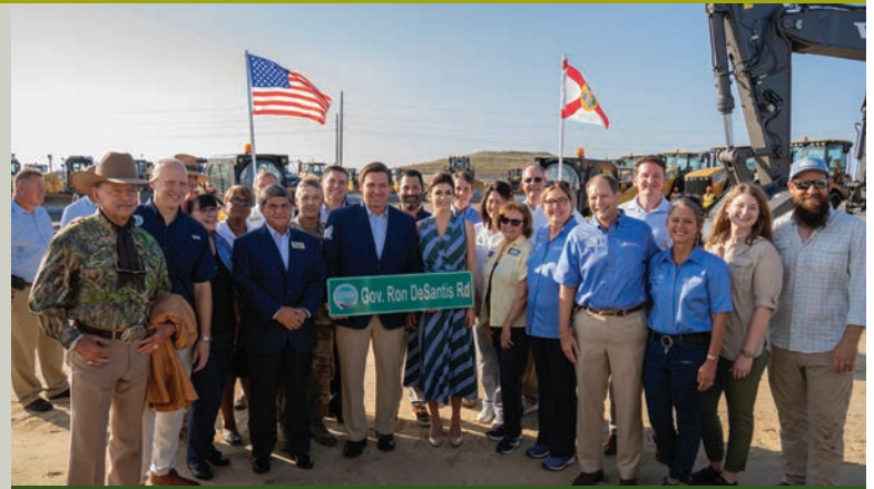
Governor Ron DeSantis, along with State and Local Officials, Breaks Ground on Embankments and Canals to Advance the C-43 Reservoir on Oct. 25, 2019. (Photo by SFWMD)
