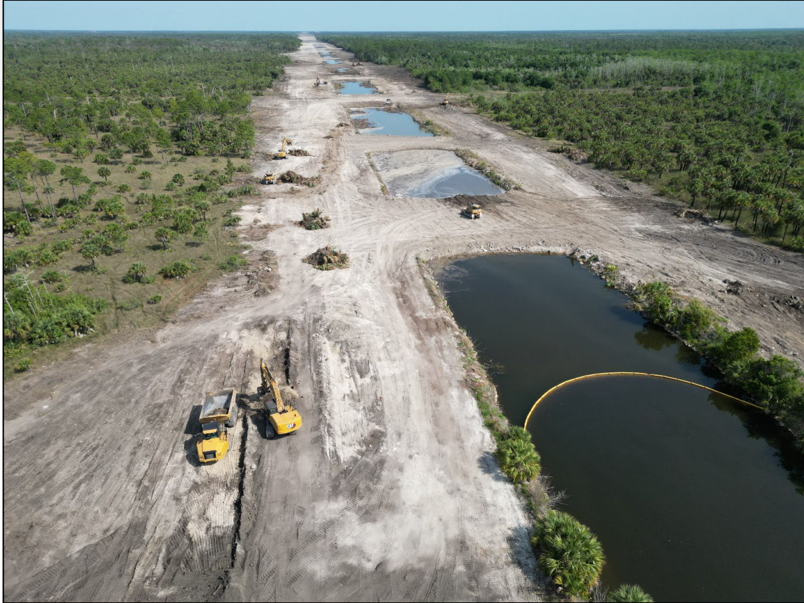
Faka Union canal backfill and clearing activities near 114 th Ave, January 2024
