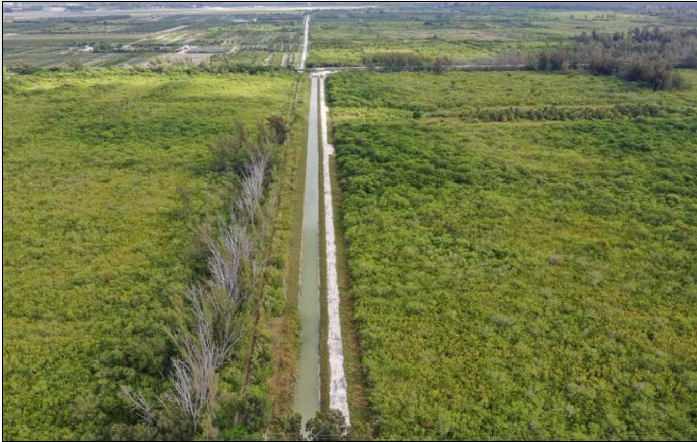
S-711 Seepage Canal, March 2024
