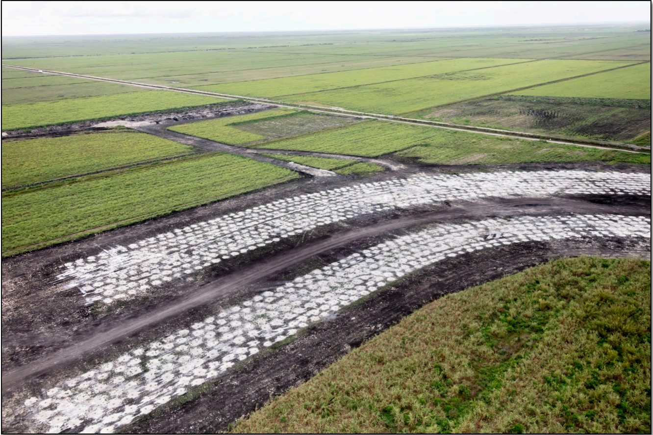
Everglades Agricultural Area (EAA) reservoir canal excavation, March 2024
