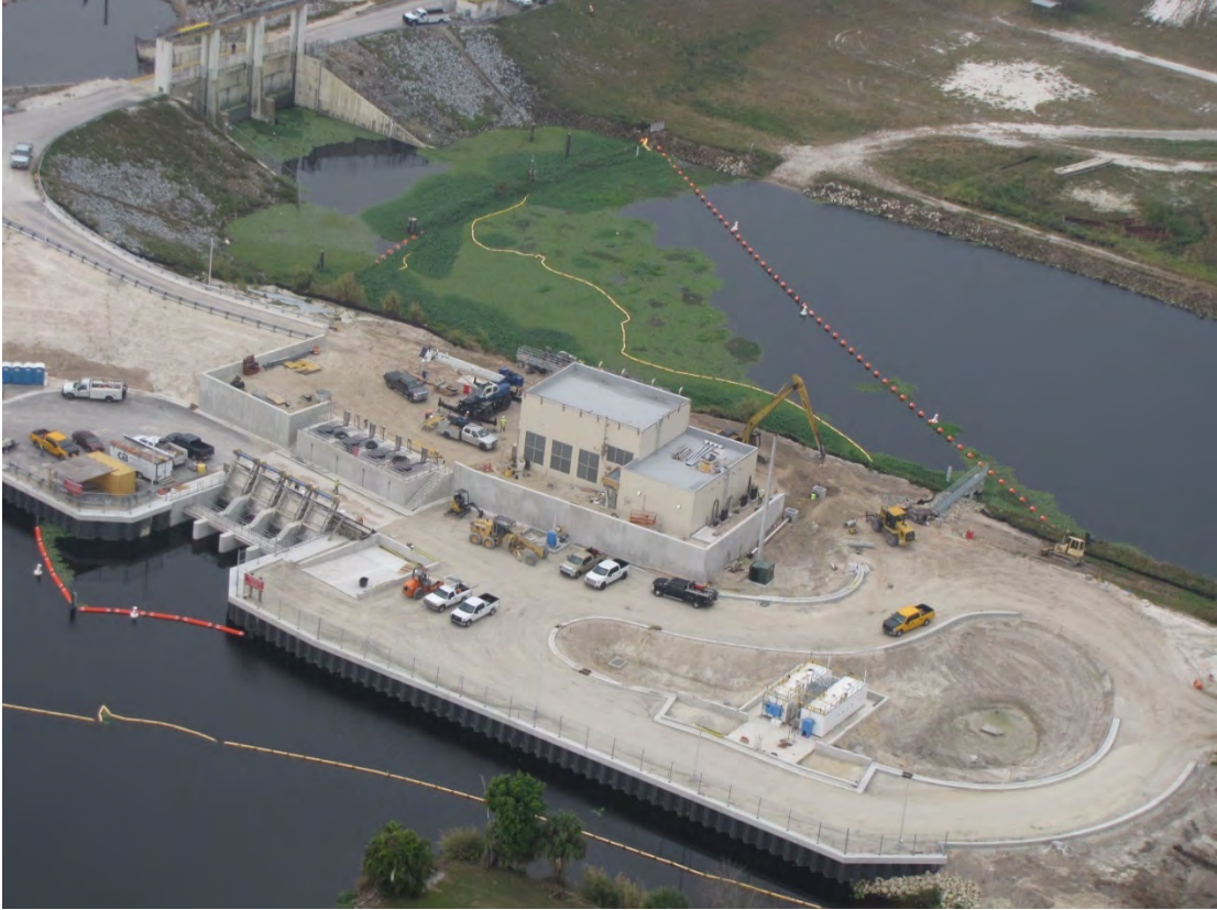
Lakeside Ranch Phase III – S-191A Pump Station Project 1515 Lakeside Ranch Stormwater Treatment Areas Page 4 of 4
