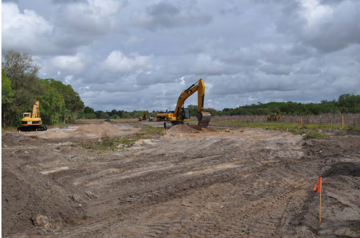
Ongoing construction of basin 4 water resource area. Photo taken March 15, 2012.
