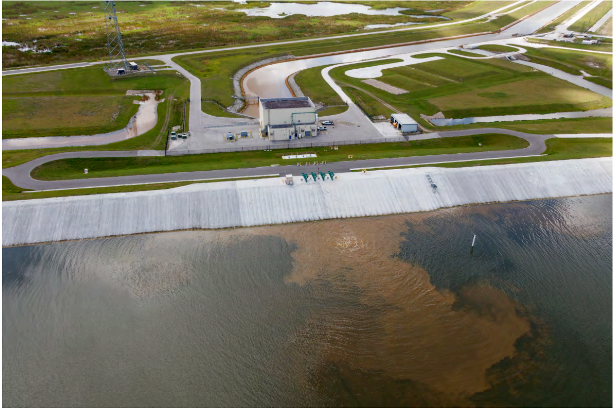
Northern view of the completed C-44 Pump Station.
