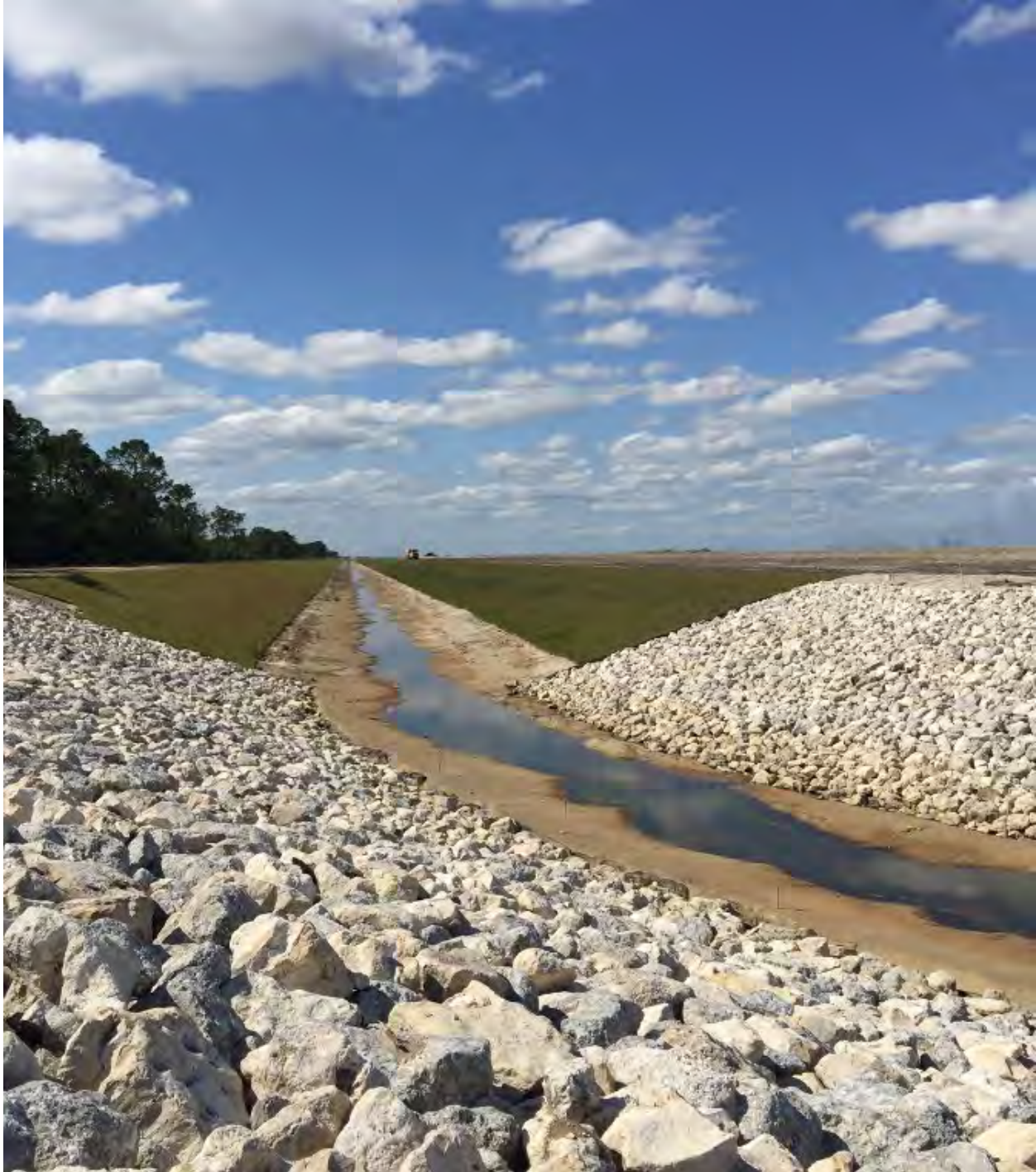
Southern view of the C-44 STA southbound collection canal from the north east corner of Cell 2.
