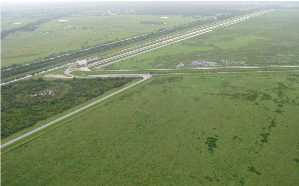
Lakeside Ranch Phase I – Northern STA and S-650 Pump Station
