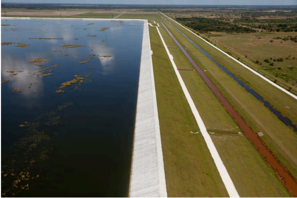
A view of the western embankment of the C-44 Reservoir.
