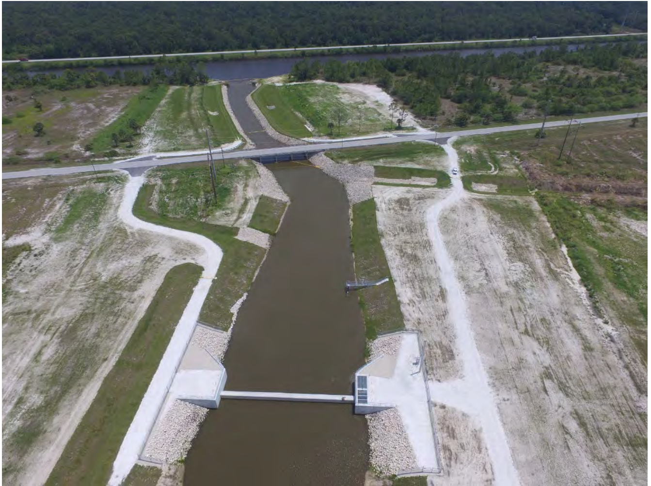
Southern view of the C-44 STA discharge canal, the C-44 System Discharge Structure S-404, and the C-44 Canal.
