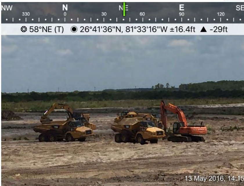
Loading fill for the Pre-load Mound
